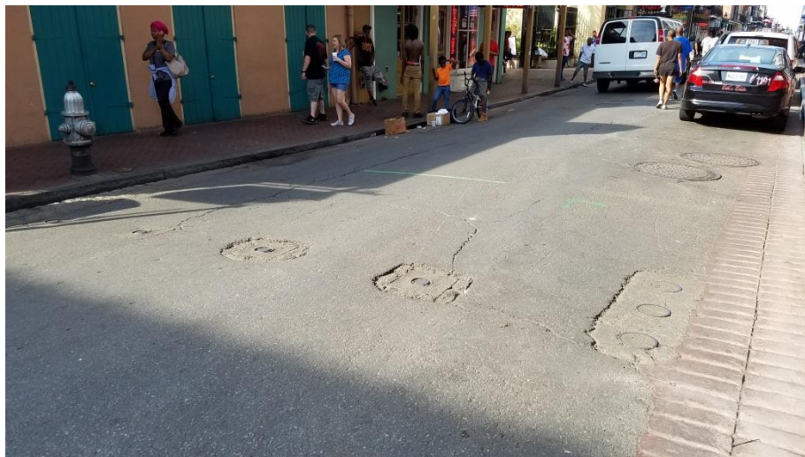
Figure 1 Existing Bourbon St Bollard Footings
